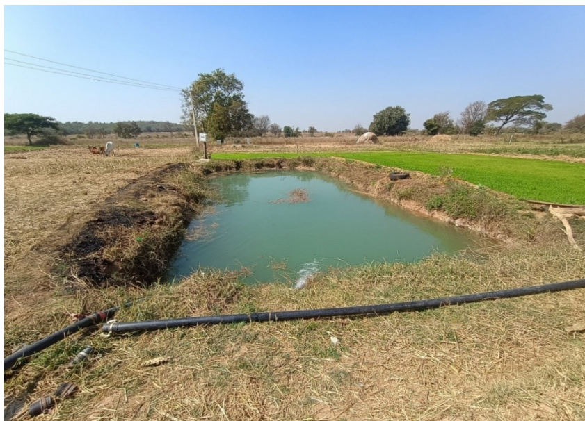
Figure 13. A seepage pond in the vicinity of Beela
