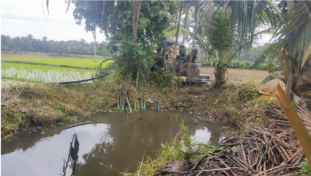
Figure 5. Typical pit at the end of a Batti channel
