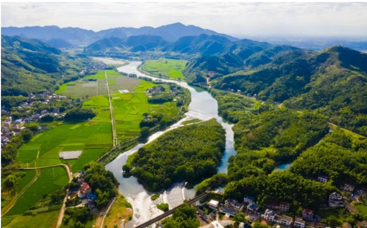
Figure 2. Aerial view of Jiang-Xi Weir
