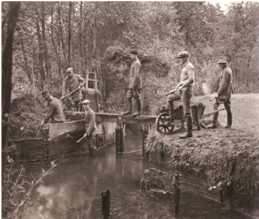
Figure 5. Meadow-irrigation students repairing a sluice gate (c. 1930) (KHG Baumgarten Collection)
