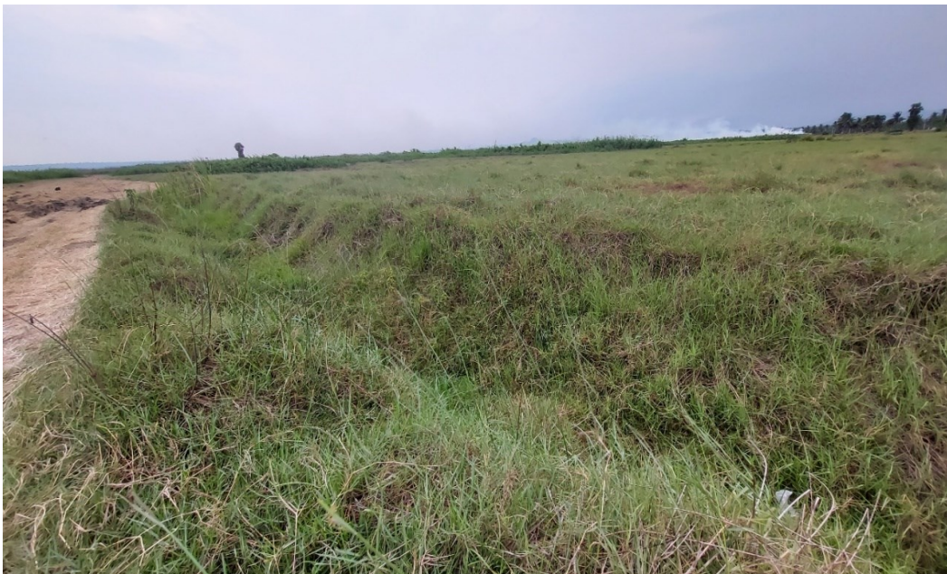
Figure 6. Dry batti channel with weed growth
